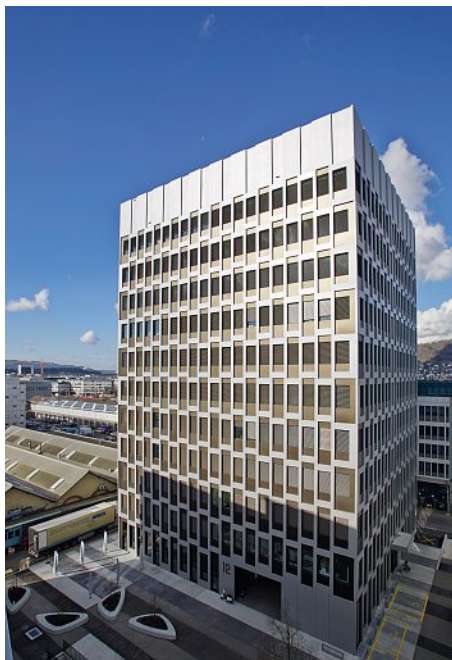
New 11-story laboratory building in the BIO-TECHNOPARK.
